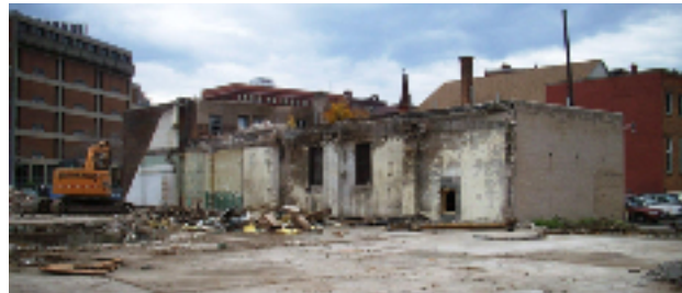
Example of a brownfield site
